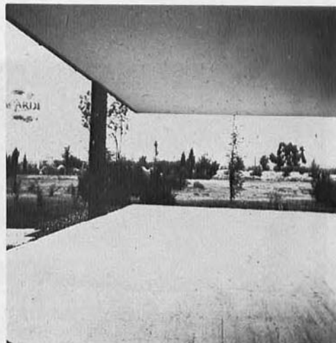
377. Bacardi Office Building, Mexico, 1961. Relation between the surfaces of floor and ceiling. Unfortunately, planting has been concentrated at the corners and will, in a few years, diminish the crystal clarity of the building.
